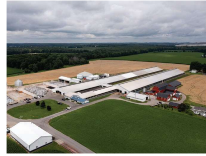
Lawnhurst Farms of Stanley, N.Y., use anaerobic digesters to convert methane, a greenhouse gas released from cow manure, into a source of electricity.
